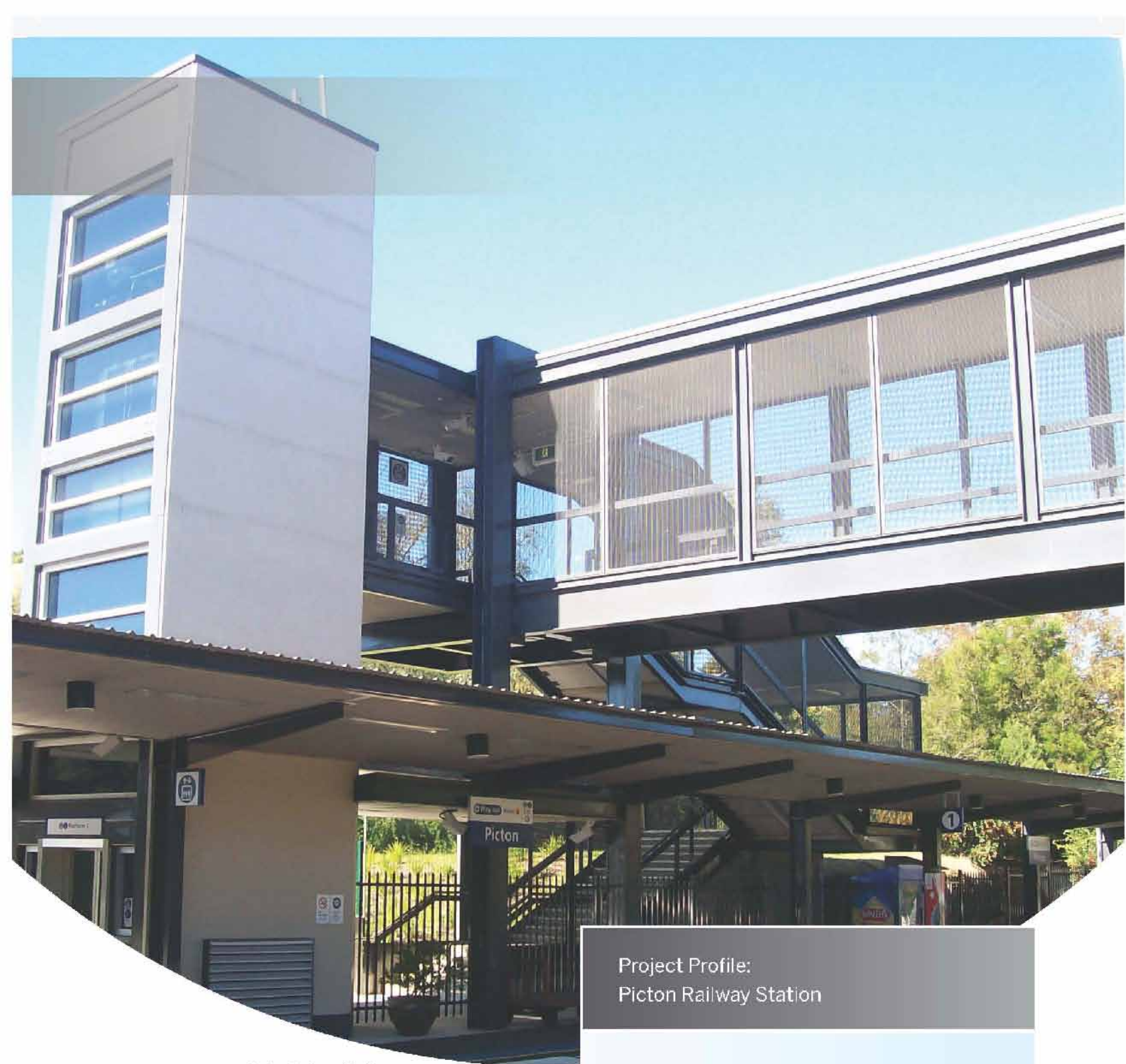
Picton Railway Station BFR ventilator
