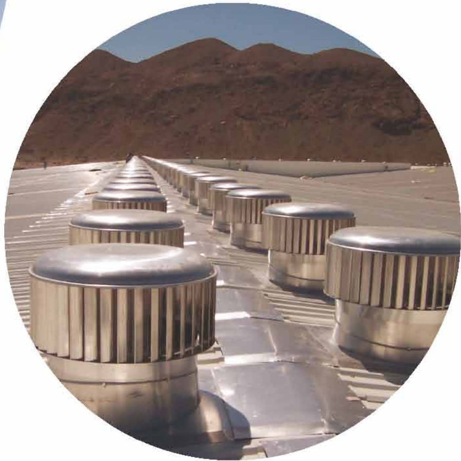
Toyota Spare Parts facility in Muscat Oman. Edmonds H900 ventilators for high ambient conditions >40°C.
